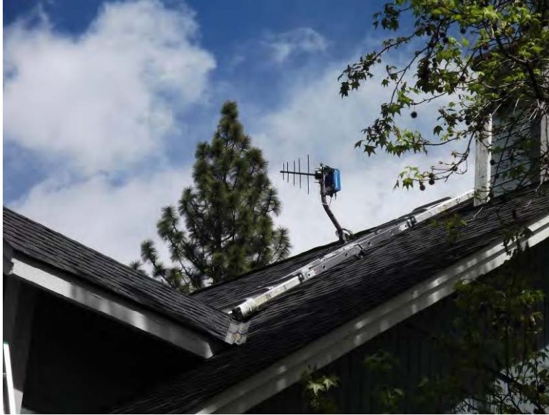
Figure 27: TV White Spaces Customer Rooftop Antenna
